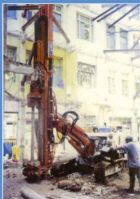
Bored Micropile Installation at Conservation House
