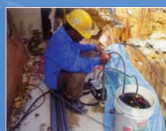
Geotechnical Instrumentation Installation & Monitoring
