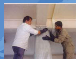
Column Strengthening by FRP System
