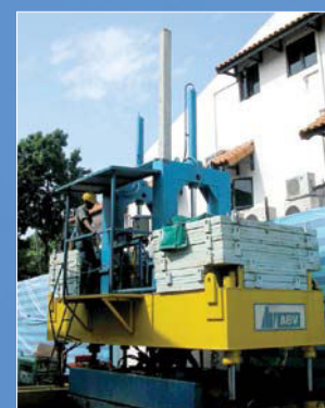
Jack In RC Pile in Residential Area
