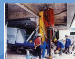
Driven Patented Steel Micropile within Low Headroom Building
